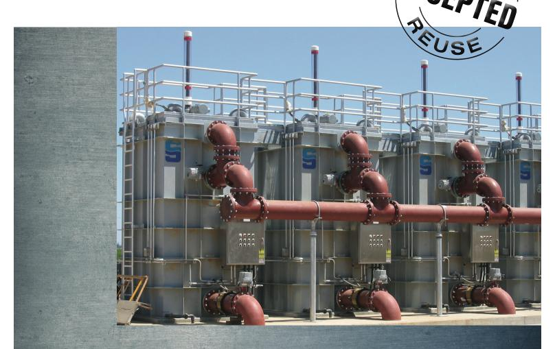
A unique innovative system for filtration rates of 40 gpm/ft<sup>2</sup>. Acceptable for water reuse under Title 22.
