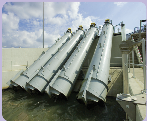
Tube Mounted Screw Pumps with a stationary outer shell eliminate the need for a precisely grouted concrete channel. Available with fixed or variable angle of inclination for control of pumping rates. Sizes from 20" to 72" in diameter. Lift capability up to 25'.
