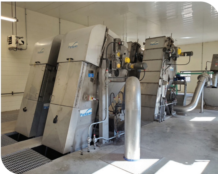
Two-stage coarse and fine screening with element screens followed by perforated screens.
