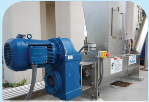
Aqua WashPress drive assembly (left) and discharge chute which connects to the Aqua Guard UltraClean (not pictured)
