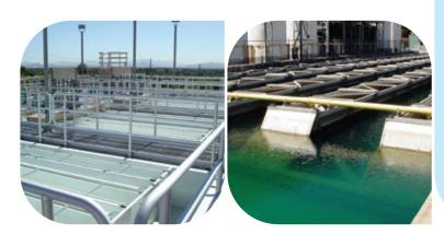
Traditional plate settlers orient the feed slots in such a way that the influent stream collides with the solids front moving down the plate to the sludge hopper. This creates a zone of interference that renders the bottom 20% of the plate area unusable for settling.
