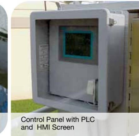
Control Panel with PLC and HMI Screen
