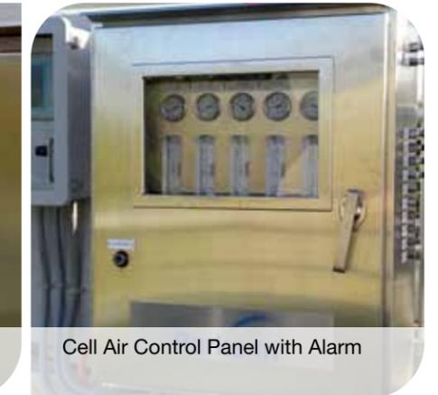
Cell Air Control Panel with Alarm
