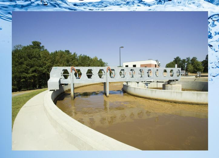
Schreiber handles sludge treatment with a unique all-in-one digester and thickener configuration.
