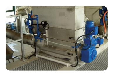
washed screenings are transferred over a barrier at one end of the wash trough into the compactor section below. The screenings are subsequently dewatered by the action of a compactor screw and conical
