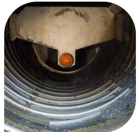
shows that rotating drum screens with perforated plates are the most successful solution for pre-membrane screening. Stringy material such as hair and lint is harmful to membranes. Unlike other technologies, Rotomesh does not allow stringy material or other types of solids to line up with screen openings and pass through.
